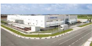
2008 - The Factory Project of Saigon Stec Co., Ltd.
