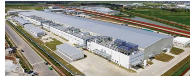
2017 - Mektec Manufacturing Corporation VN New Factory Project
