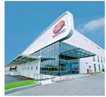
2018 - Dan On Foods Corporation - My Phuoc 3 Branch New Factory Project
