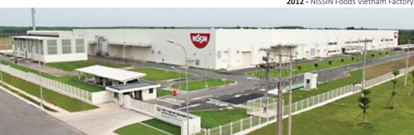
2012 - NISSIN Foods Vietnam Factory
